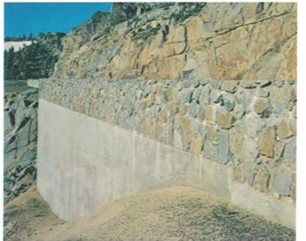
Rock masonry on poured concrete. If the entire retaining wall were composed of rock masonry, it would blend well.
