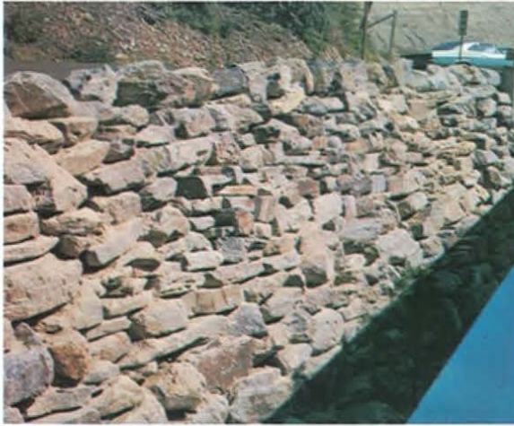
Dry wall of large rock
