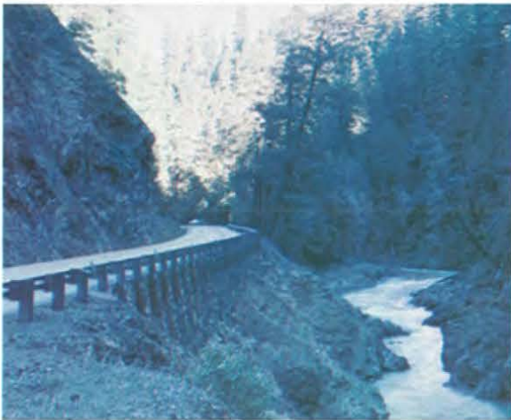
Rock masonry with guardrail
